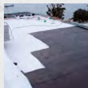
Waterproofing on bitumen
