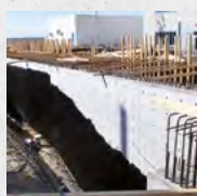
External basement waterproofing
