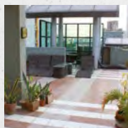
Waterproofing balconies / terrace
