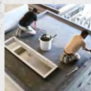
Precast concrete production
