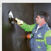
Waterproofing against Radon
