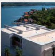
Liquid roof waterproofing
