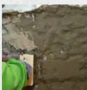
Internal basement waterproofing
