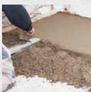
For creating a waterproof screed
