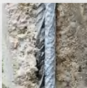
Corrosion protection (coating)
