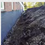
External basement waterproofing
