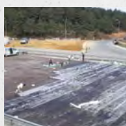
Floor slab waterproofing
