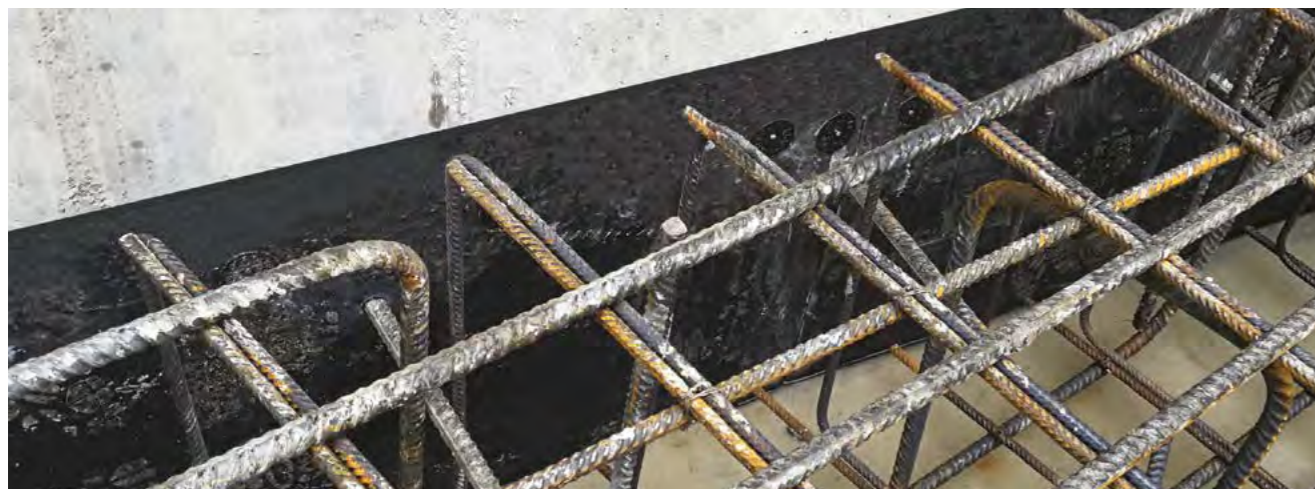
Application of hydro-expanding rubber joint panel type R for concrete slab sealing
