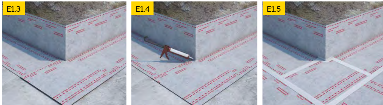
E1.1/E1.2/E1.3/E1.4/E1.5 Sealing of internal 90° corner on formworks
