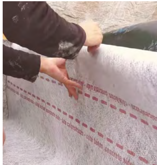
90° corner in case of open basement excavation with Delta Amphibia system
