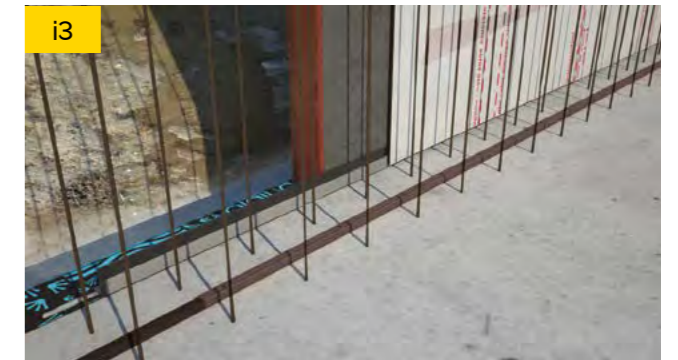
i1/i2/i3. Construction joint with Delta Amphibia pre-applied on formworks with toe
