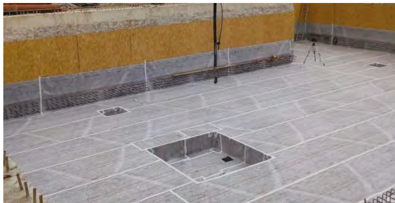
Lift pit with Delta Amphibia system
