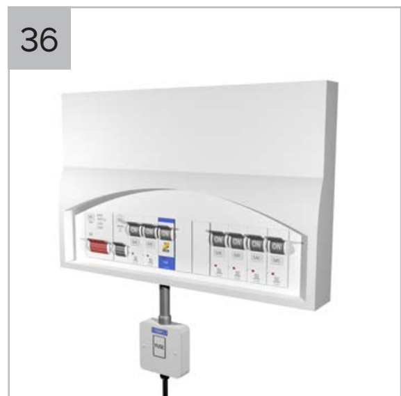
36 Isolate main supply and connect the pump to a separate non-switched fused spur. When installing a Delta HLA, follow the wiring diagram on page 18.
