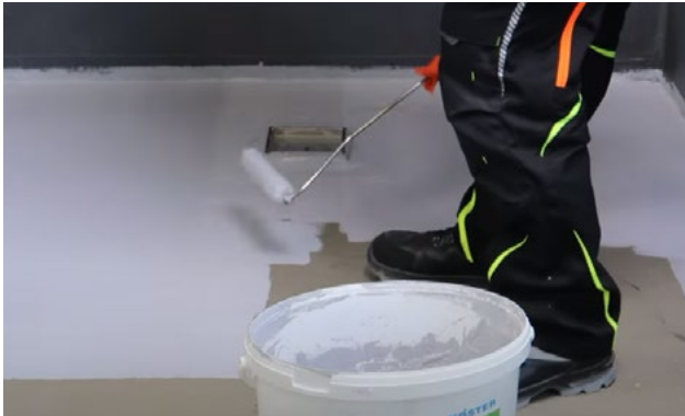
1st layer on the floor
