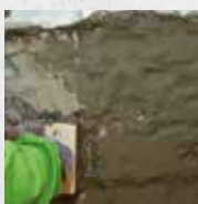
Internal basement waterproofing
