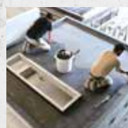
Precast concrete production
