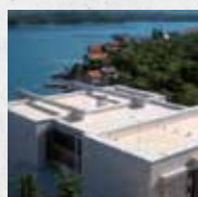
Liquid roof waterproofing
