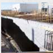
External basement waterproofing
