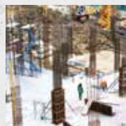
Applicable to concrete after 7 days
