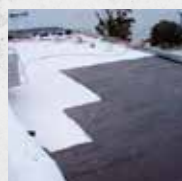
Waterproofing on bitumen
