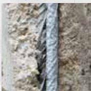
Corrosion protection (coating)
