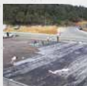
Floor slab waterproofing
