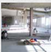
Restoration of support beams
