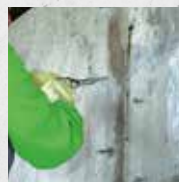
Forms resin in dry cracks
