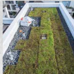
Under ballast / green roofs
