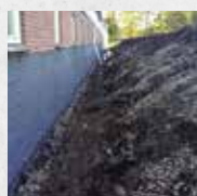
External basement waterproofing
