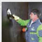
Waterproofing against Radon
