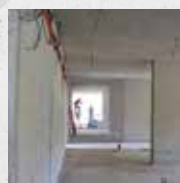
Large surface restoration
